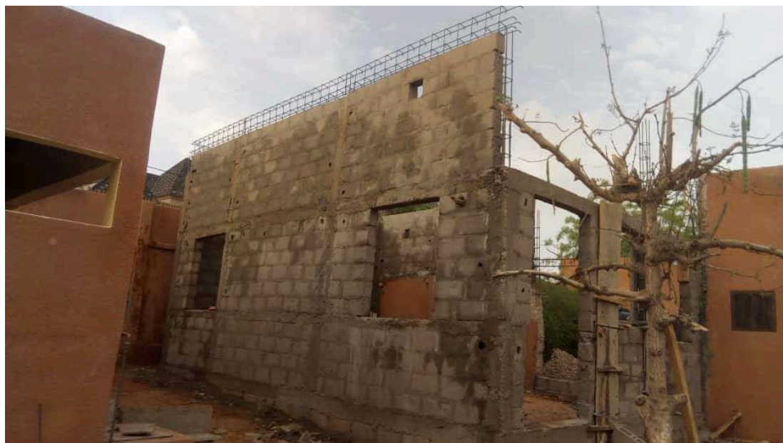
The kindergarten room under construction – March 2020
