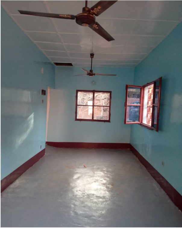
Infirmery Addition, June 2020
