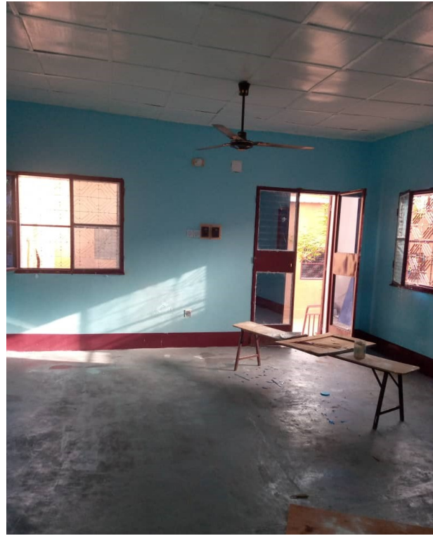
Inside the new kindergarten building
